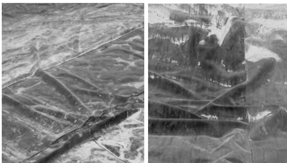
FIGURE 8 - Elongation of geomembrane due to shape deformations based on climatic conditions.
