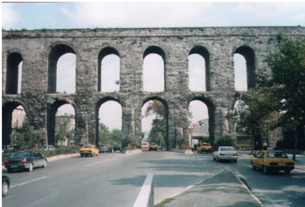
Figure 3. A general view of the Bozdogan (Valens) aqueduct (by authors).
