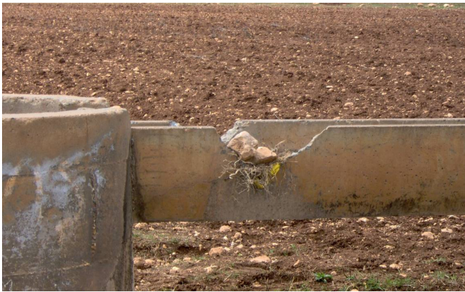
Figure 3. Taking of water by breaking the small channels.
