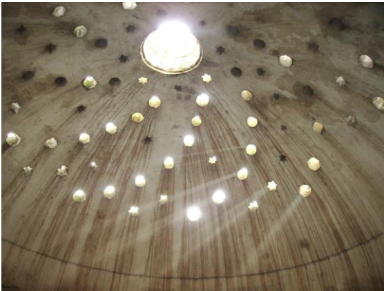
Figure 3. The interior view of Yalınayak Bath, Tire-Izmir, Turkey (Reyhan et al., 2013)
