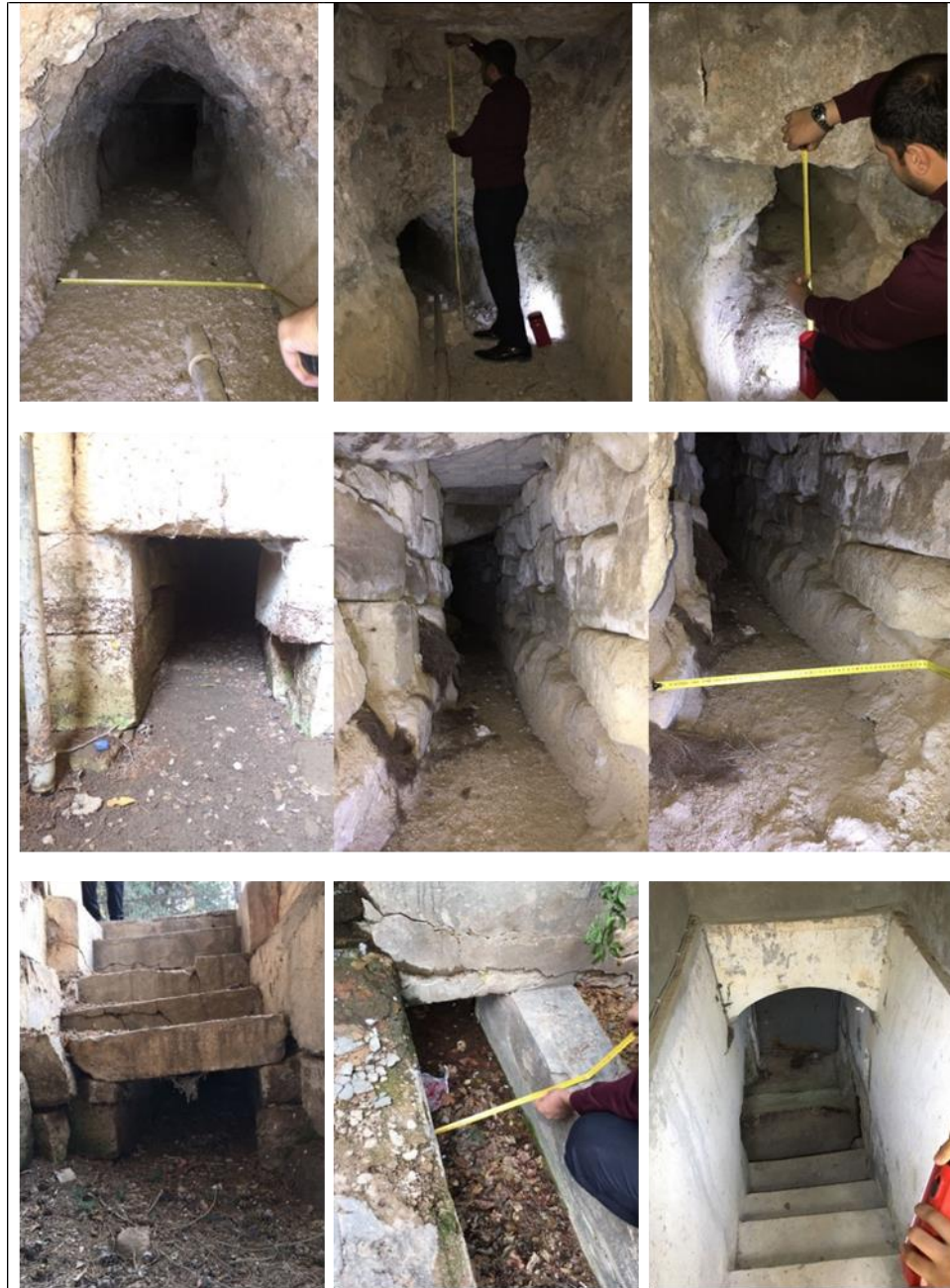
Figure 6. The details of kehriz galleries of Little and Middle Springs of Germüş Water; Views of Circular Galleries and Stone Braid Walls of Tunnels, from Site Study of the Authors.
