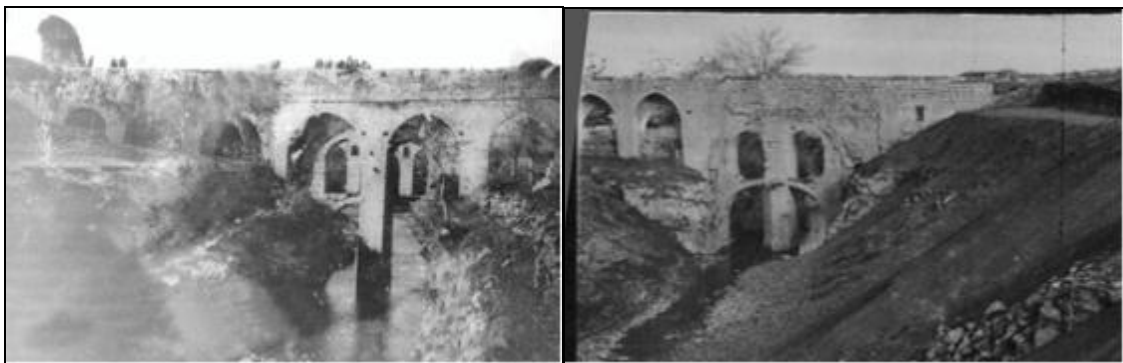
Figure 16. Old views of Karakoyun (justinian) Aqueduct (C. Kürkçüoğlu archive)
