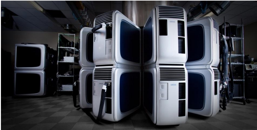
“Sneak Peak: Inside NVIDIA’s Emulation Lab” – http://blogs.nvidia.com (Cadence Palladium cluster used for GPU emulation)
